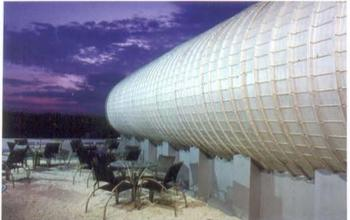
For Tube we hit upon the idea of an elliptical lounge space, with a cross-section like an aircraft. This was to straddle the terrace and shout its presence on the street, much like an architectural billboard. Constructed out of tubular steel hollow sections with a galvanized sheet roofing skin, it was clad on the inside with soft faux leather quilting. We inserted a dance floor in the centre, along the spine and put laminated glass as flooring that provided view of the terrace 3' below.
